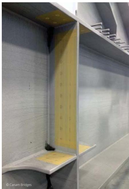
**Figure 1 (left) - The liquid zinc solidifies in contact with steel and it creates a coating with a thickness between 20 and 300  $\mu\text{m}$ .**
